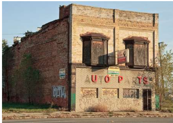
Figure 10.3 This dilapidated auto supply store in Detroit is a victim of auto industry outsourcing. (Photo courtesy of Bob Jagendorf/flickr)
