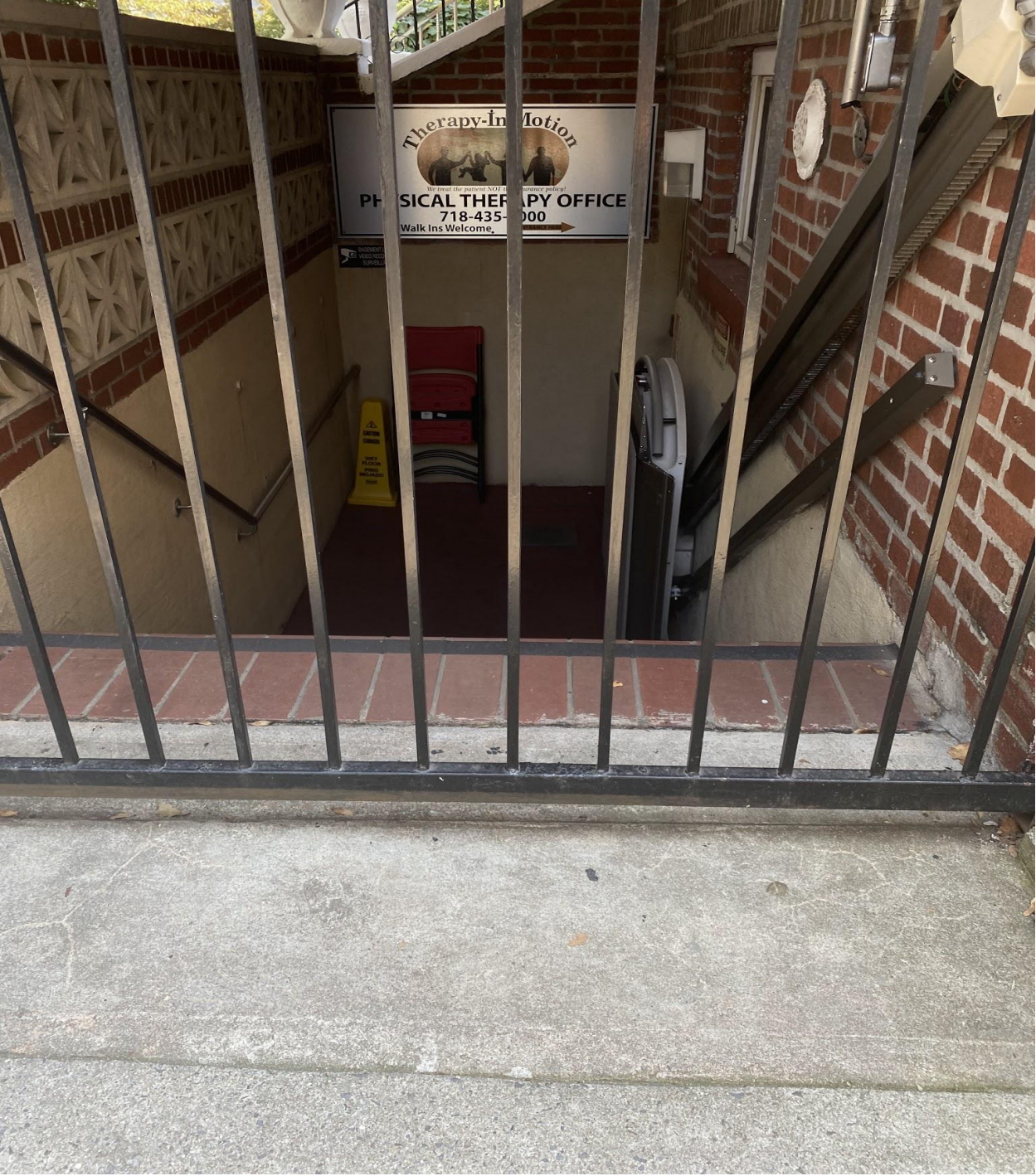
This picture shows the mechanical ramp for people with special needs.
